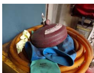
圖 7-2 感溫型滅火器因鏽蝕 脫落 Automatic fire extinguisher fell off
